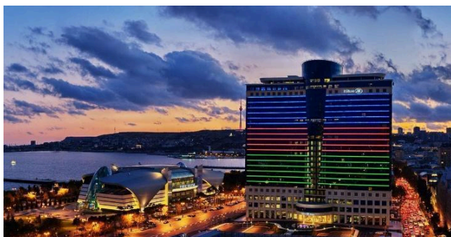
Building 1: 1B Azadlig Avenue Rooftop Bar Sky Grill, Hilton Hotel
