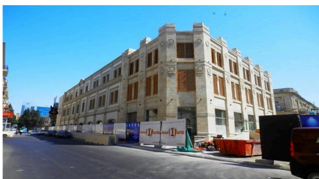
Building 2: 8, Aziz Aliyev Street. Roof of the Cinema Plus Building
